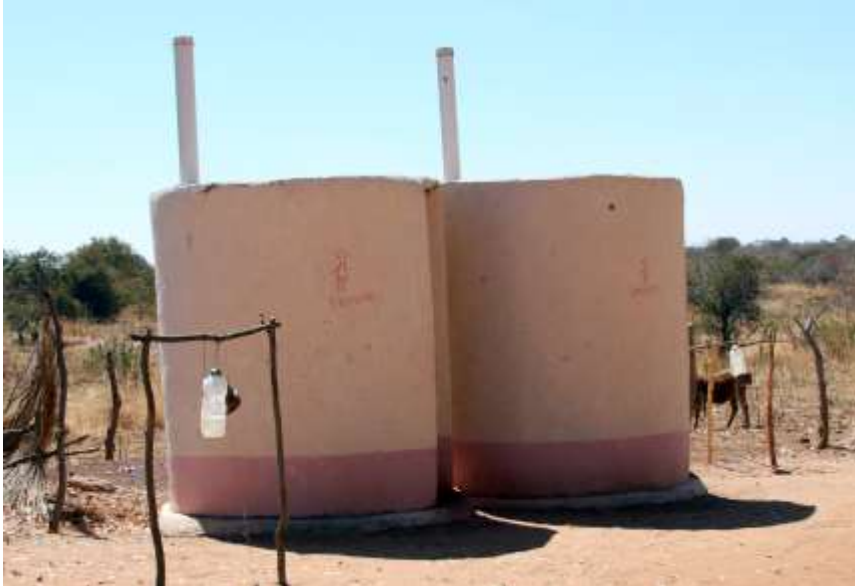
Improved, ventilated latrines, constructed with the proceeds of vegetable sales
